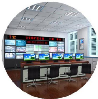
CCTV Security Transmission
